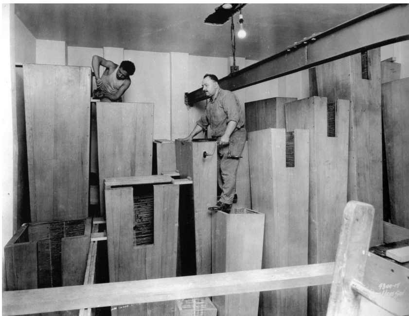
Figure 14. Building the 32-foot Diaphone, Atlantic City
